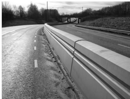
Figure 5.8 Single slope barriers
