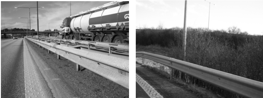
Figure 5.3 Figure W-beam barriers
