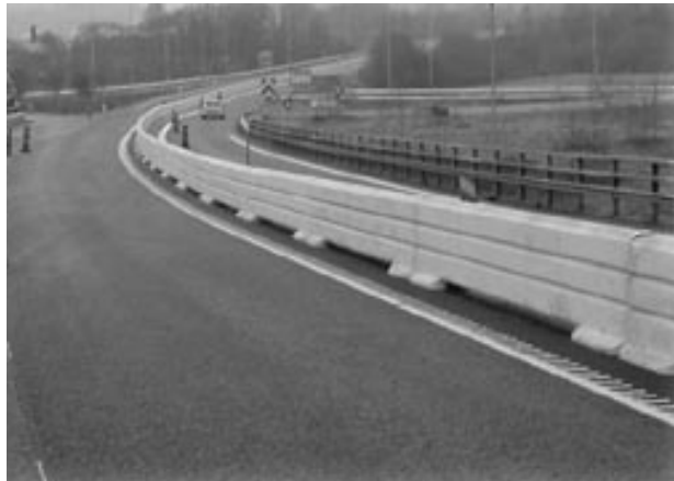
Figure 5.9 Vertical concrete barrier (GP-LINK)
